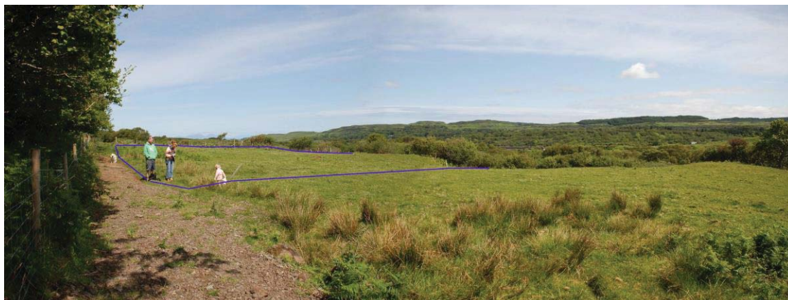
Photograph 1: Photo from Building Warrant submission showing the access track in place.
